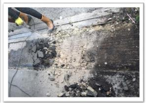
The outcome: With all concrete defects to the relevant car park decks and entrance repaired, the lines of which the defunct cathodic protection had started to come through the surface of the deck have been removed and now repaired and protected. The addition of the interdeck coating also guaranteed enhanced protection from further degradation to the concrete surfaces. The works completed ensured the Mayorhold multi-storey carpark was successfully repaired and reinstated.
