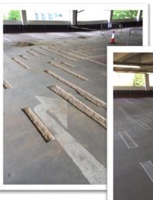
instating new white lining and symbols, ensuring it matched the existing profile. Repairs to the car park entrance were also required, with the existing defective asphalt first removed, followed by the preparation of the concrete
