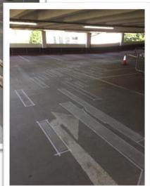
surface. Reinstatement was carried out using Sika Rapid Repair mortar as well as the application of a Tremco anti-slip coating.
