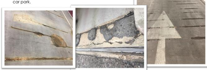
**The solution:** With repairs focussing on levels 2, 3 and 4 of the car park, all areas of defective concrete slabs were first broken out using a pneumatic drill, with any exposed cabling and mesh strips cut away and discarded. Once the areas were adequately broken out to a sufficient depth, cleaned and primed, they were repaired using Sika Rapid Repair Mortar. A rapid cure Tremco interdeck system was then applied to the repaired deck area, before re-
